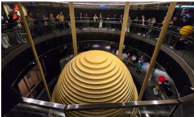
Photo of the Taipei 101's 660-tonne gold-colored tuned mass damper swings like a giant pendulum between floors 87 and 92, stabilising the skyscraper against typhoons and earthquakes.
